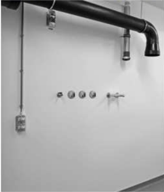
Project: Hospital operating theatres and other facilities | Installation: PALOPAQUE™ HYG White with welding rods
