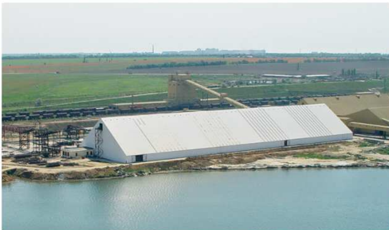
Project: TIS Port - Odessa, Ukraine | Type: PALRUF® 3mm White Opaque and Clear (Clear sheets used as skylights)
