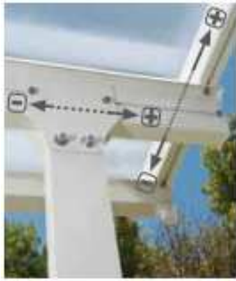
Position adjustment of poles
